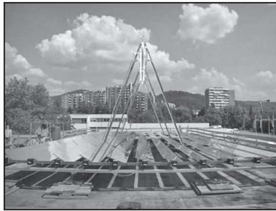
The PSE Fresnel collector installed on the rooftop to power a NH 3 /H 2 O absorption chiller (Source: PSE, Germany)
