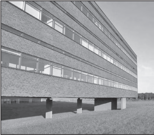
The north and south facades of the Bang & Olufsen Headquarters in Denmark. B&O's building is an energy efficient building with good daylight, natural ventilation, and only the north facade is completely glazed. (© Steen Traberg-Borup, The Danish Building and Urban Research)
