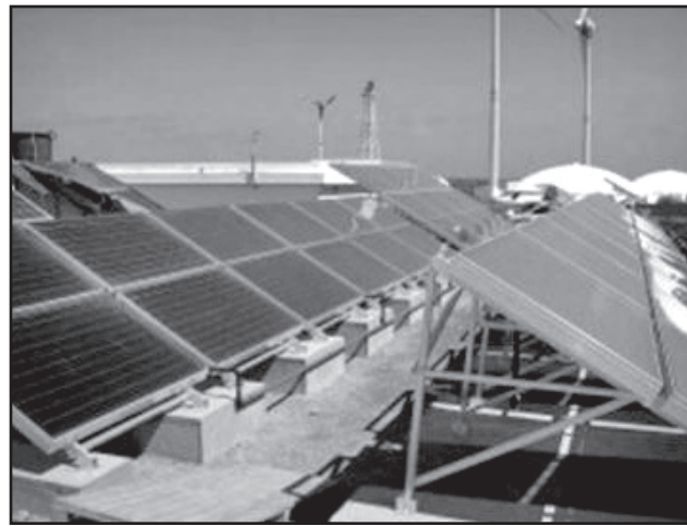
Sea water desalination in Gran Canaria, Spain (Fraunhofer ISE, Germany).
