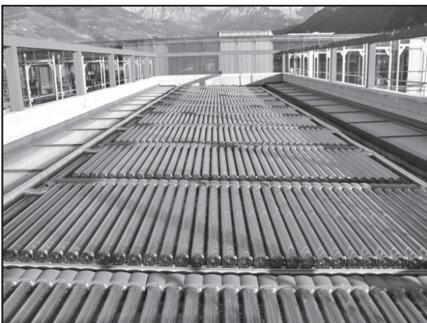
Solar collector field of the solar cooling system at European Academy in Bolzano/Italy. The first expert meeting took place in this building.
