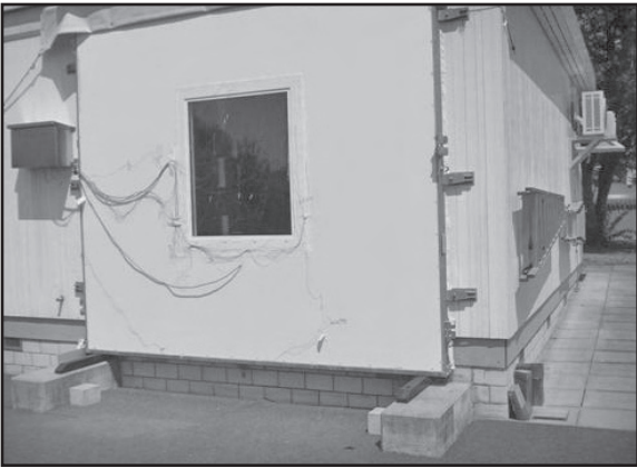
EMPA Test Cells in Duebendorf, Switzerland
