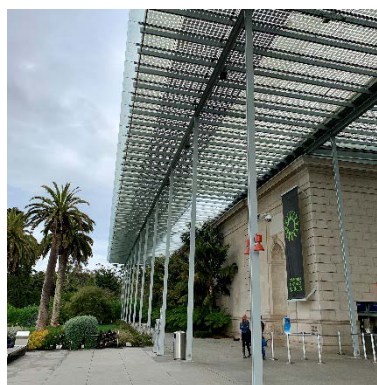
Photovoltaic shelter - California Academy of Science, San Francisco (USA) Photo: M. Formolli
