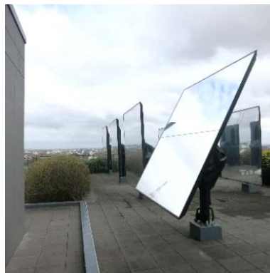
Heliostat mirror - One Central Park, Sydney (Australia) Photo: M. Snow
