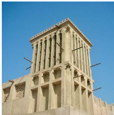
Wind tower - Dubai (United Arab Emirates) Photo: M. Formolli
