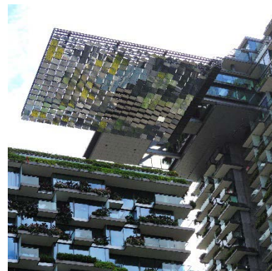
Cantilevered reflector system - One Central Park, Sydney (Australia) Photo: S. Croce
