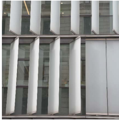
Vertical louvres applied on an office building - Vienna (Austria) Photo: S. Croce
