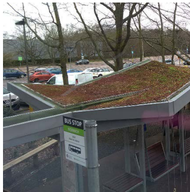
Vegetated bus stop - Norwich (United Kingdom)
