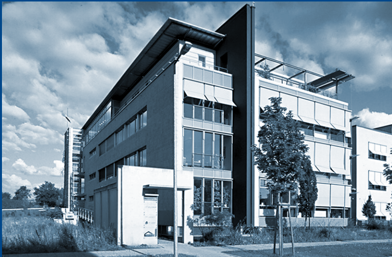
Figure 1: High quality integration of building structure and energy system in an architectural concept will also determine the aesthetics of a building: the WAT office building in Karlsruhe, Germany, synchronises both structural and energy purposes by means of a "black wall", which combines several functions in a single unit: a glazed solar chimney in a two-storey core atrium acts as a solar-driven engine for the ventilation system. It also contains service pipes, feed lines and installation systems for the purposes of structural stiffening. The WAT office building is documented by the IEA Task 23 Case Stories collection.
