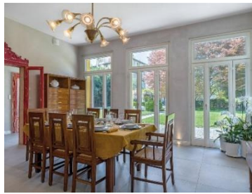
Figure 29: Villa Castelli . Old windows replaced by similar new ones.
