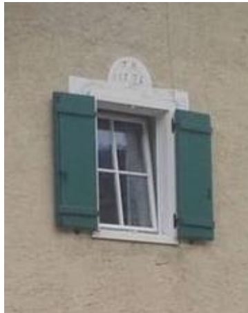
Figure 40: Oberbergerhof. Thin frame with a historic appearance.
