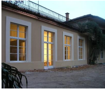
Figure 36: Ansit Kofler. Façade restored to original state.
