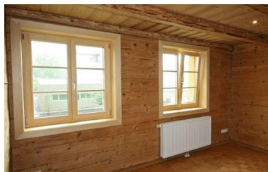
Figure 43: Baur Residence, Lustenau. Windows moved back to original place
