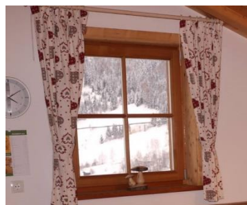
Figure 31: Obergasserhof . Single-leaf and double-glazed new windows.
