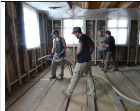
Figure 3: timber framed house in Alsace, sprayed hemp concrete
