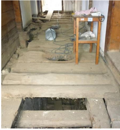
Figure 21: Aussergrubhof, old wooden floor joists
