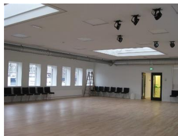
Figure 27: Osramhuset . New roof windows increased daylighting levels.
