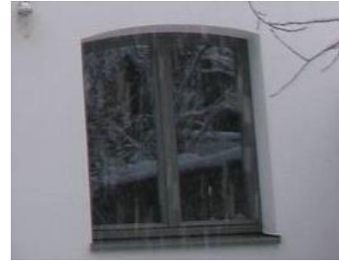
Figure 38: Maison Rubens. New oak wood windows.
