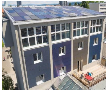
Figure 66: Solar Silo . Coloured customized photovoltaic modules creating a particular visual design.
