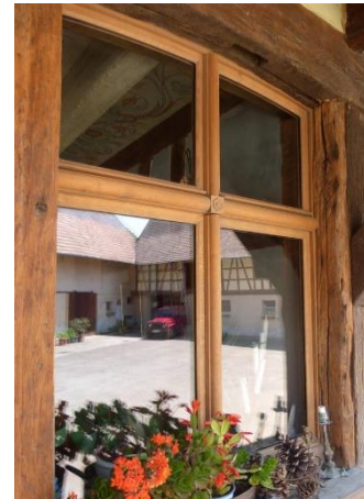
Figure 41: Timber-framed house in Alsace. New double-glazed solution.
