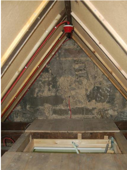
Figure 12: Hollyrood Park Lodge, pitched roof with wood fibre
