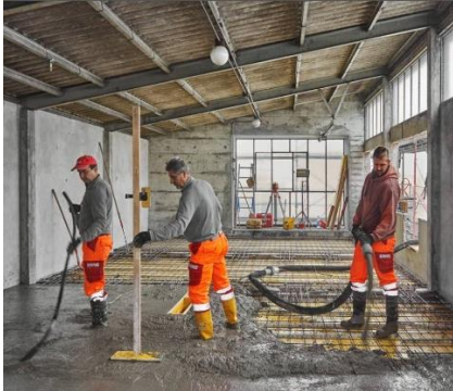
Figure 15: Solar Silo, old beam structure
