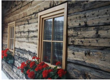
Figure 33: Aussergrubhof . Larch wood double-glazed windows.
