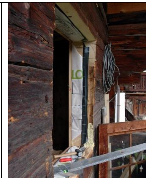
Figure 5: Aussergrubhof, internal hemp fibre insulation
