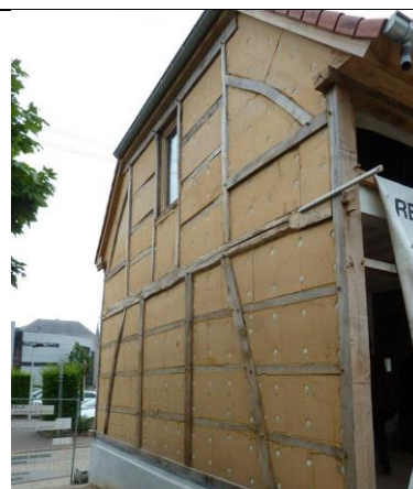
Figure 7: half-timbered house in Alkjen, wood fibre board with clay plaster
