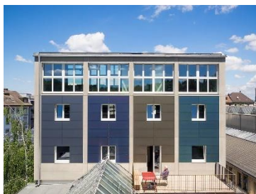
Figure 26: Solar silo . New windows added to the façade.
