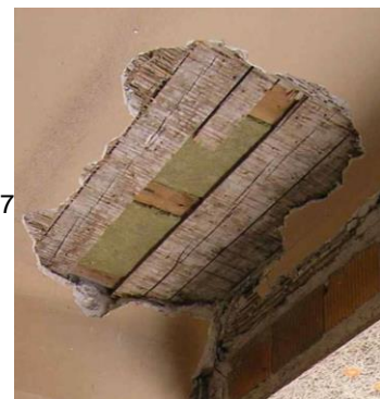
Figure 11: Ansitz Kofler, bottom view of the insulation between the rafters
