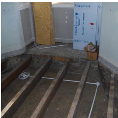
Figure 18: Hollyrood Park Lodge, suspended timber floors
