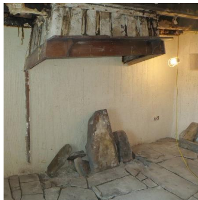
Figure 19: Downie's Cottage, original flagstone floor
