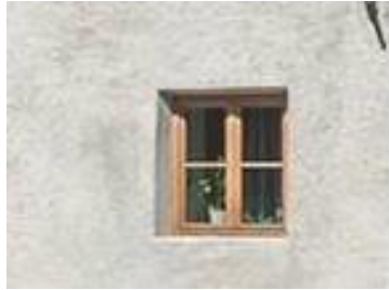
Figure 34: Ruckenzaunerhof . New windows selected in close cooperation with monument office.
