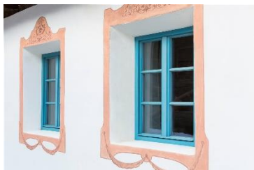
Figure 42: Rainhof. Windows produced by local furniture maker.
