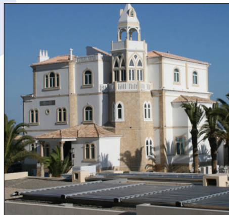
◀ Figure 7. Collectors used for hot water preparation and swimming pool heating at the Bela Vista Hotel and Spa in Paria da Rocha
