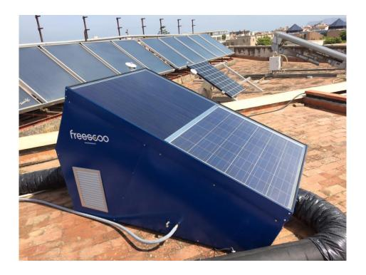
The system is composed by a solar photovoltaic/thermal air collector, two adsorption beds, an integrated cooling tower, two wet heat exchangers, fans, batteries and all other auxiliaries needed to perform the air handling process also in stand-alone operation. During winter, if solar radiation is available, warm air can be delivered to the building.
