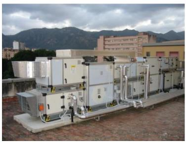
Air handling unit desiccant cooling (AHU-DEC)
